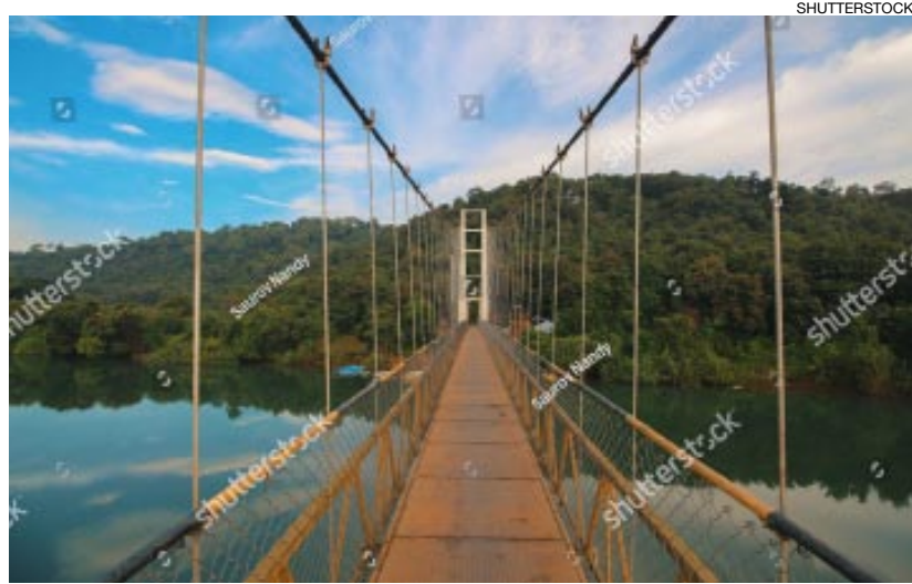
A narrow suspension bridge over river Sharavati
