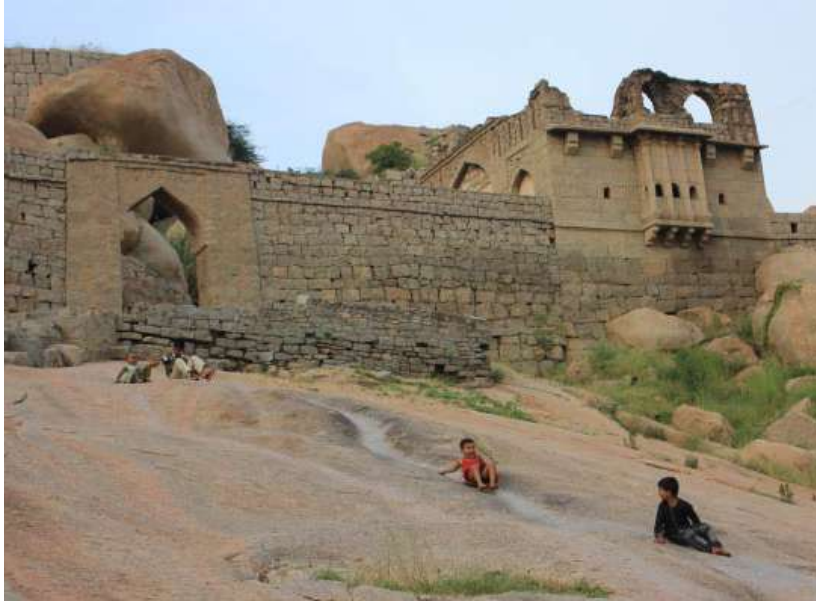
Ballari Fort, whose faulty renovation led to a death sentence for a Frenchman
