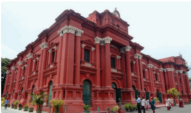
The Government Museum building was constructed in 1877
